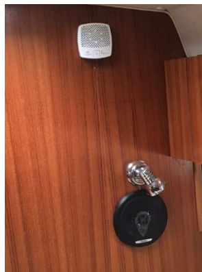
Align holes and rotate detector slightly clockwise to attach CMD5 alarm
